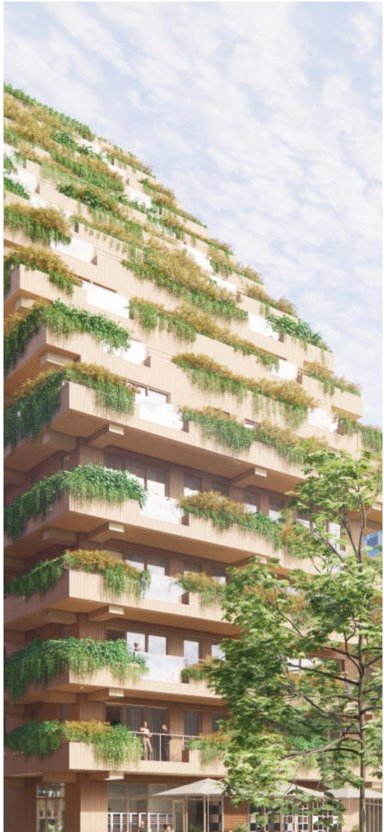
SAWA, “the healthiest building in The Netherlands” and Rotterdam’s first wooden residential high-rise - designed by Mei - makes extensive use of cross-laminated timber (CLT). Image courtesy of Mei
